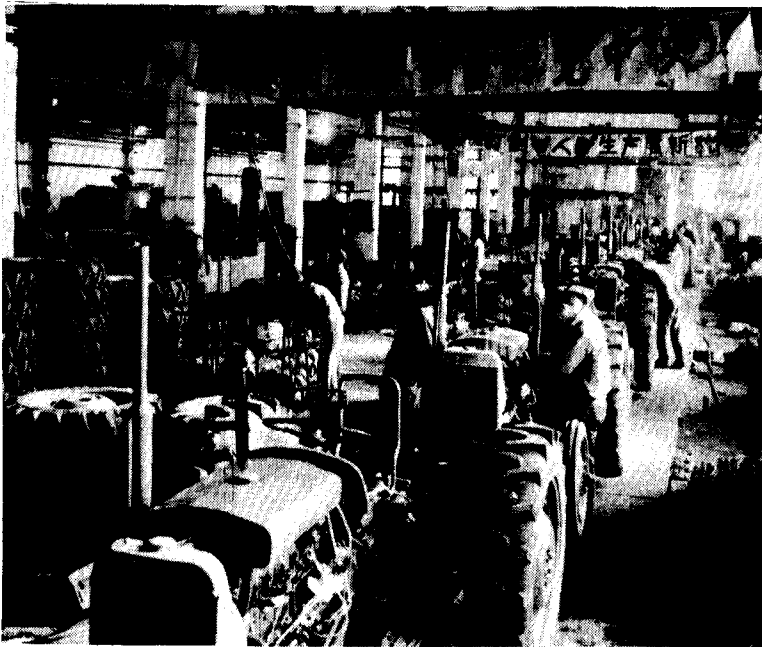
The plant is now in full operation.
